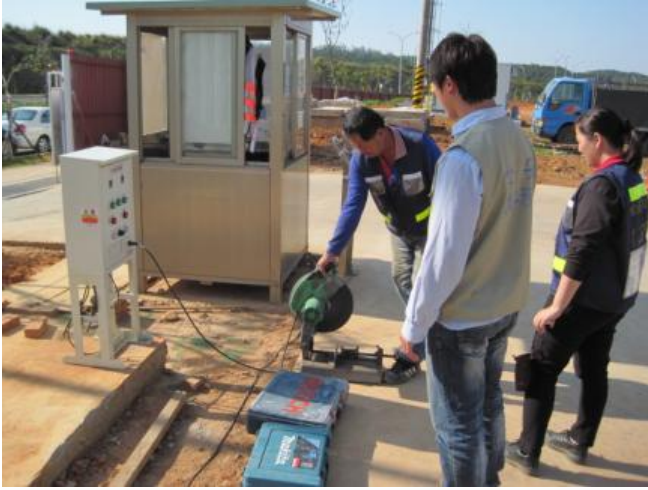
Appliance equipment performs power leakage test and is immediately quailed.
